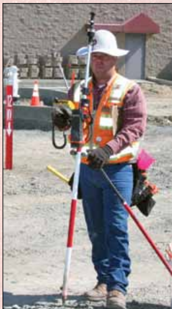
uck Brooks with ific stakes grade for gutters on the 49ers project in Santa Clara.
