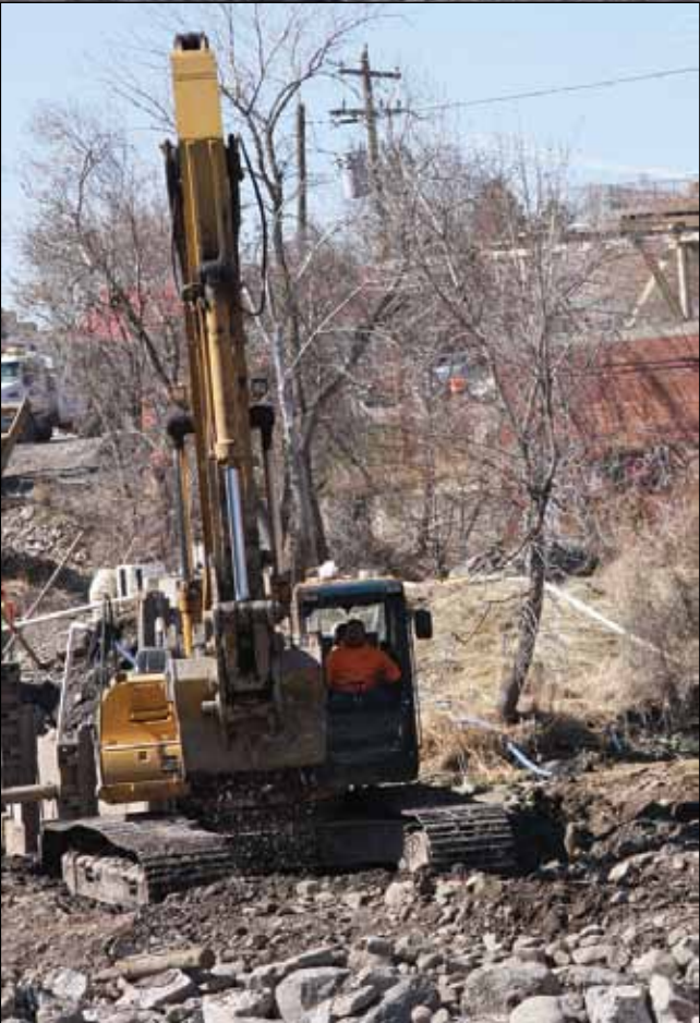
Josh Richins uses a grizzly bucket to screen native material back onto the riverbank.
