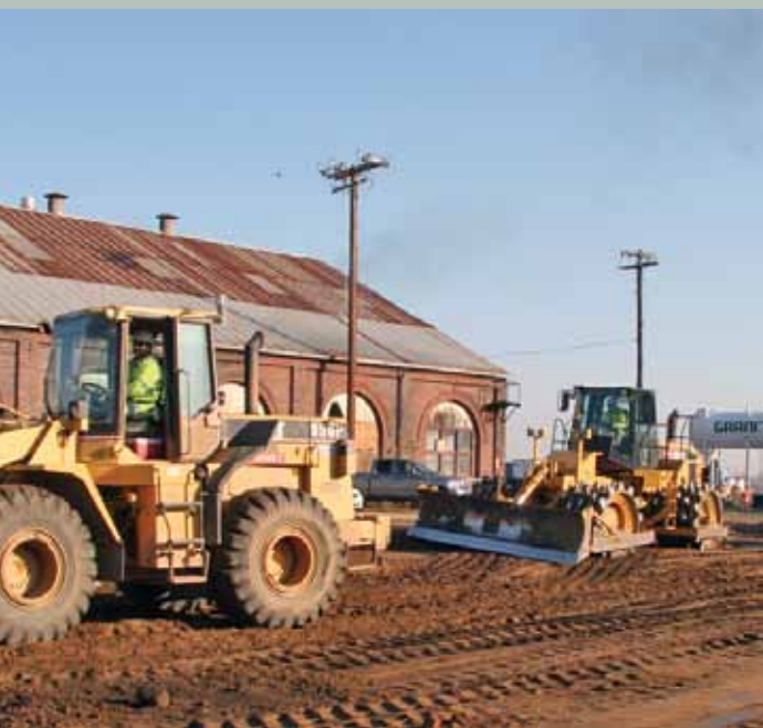
Compactor Operator Robert Magana work together to fill and level the area behind a brick building that will eventually be preserved for adaptive reuse.
