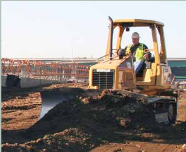
Dozer Operator Matt Barker fills and levels the area around one of many tunnels on the Sacramento Railyards project.
