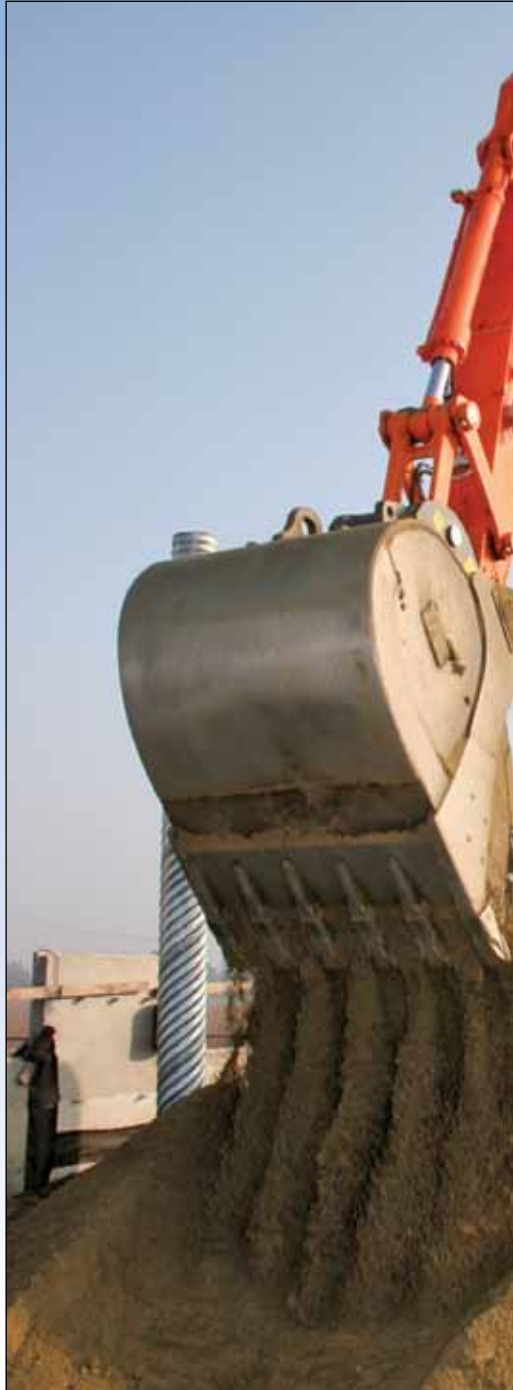
Excavator Operator Kurt Milovich mixes material that will be used on the MSE walls.
