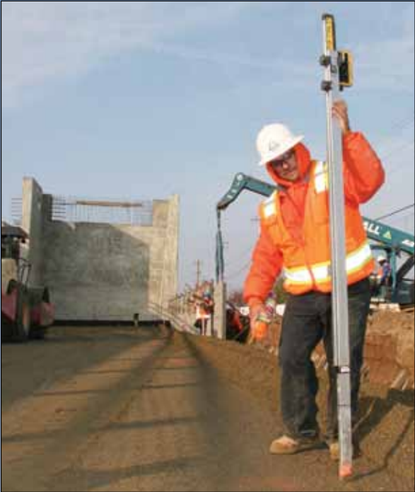
Gradesetter Tony Reyes helps bring up the fill on the Hwy. 140 ramp.
