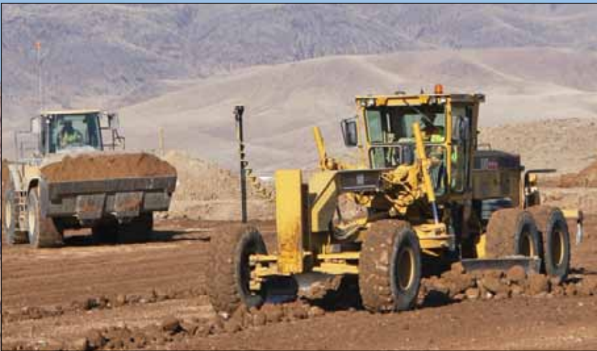
Loader Operator Jeff Glass and Blade Operator Travis Kincade take the pad to finish grade.
