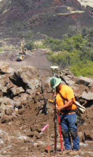
Gradesetter Francis Ke sets stakes for Dozer Operator Abraham Kihe, as crews cut a new road for the WB Kukio Stroud subdivision job that involves a steep, 20 percent grade.
