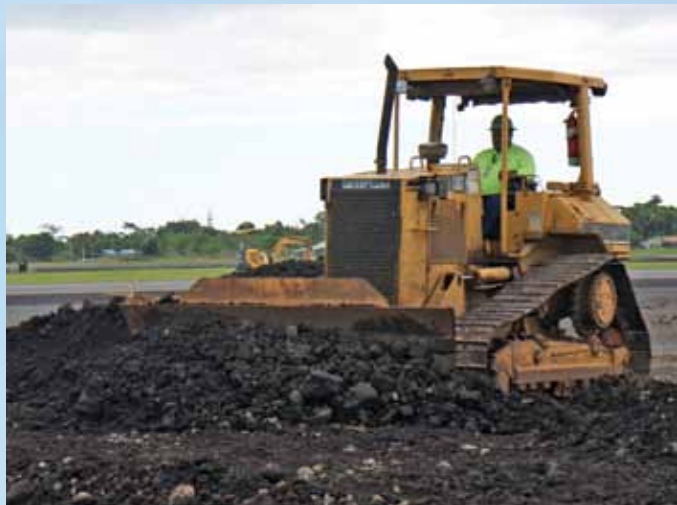
On the Hilo Airport project, Steven Uemura preps a taxiway for subgrade.
