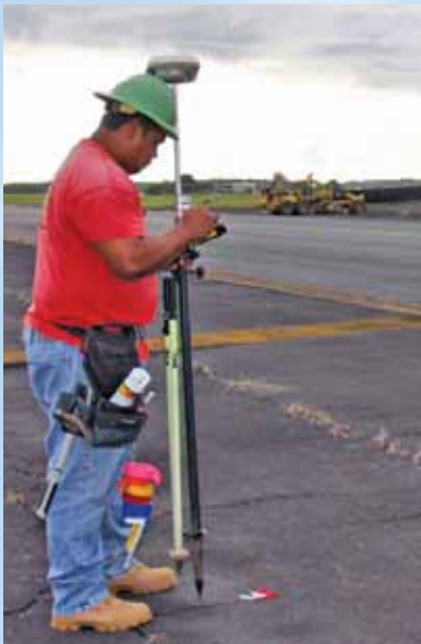
Gradesetter Dwight Enriquez sets points for runway lights on the $28 million Hilo Airport project.
