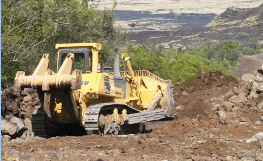
Member Hauoli Hanohano works on the WB Kukio Stroud subdivision project, which entails a half-mile of mass grading for a road and a waterline.
