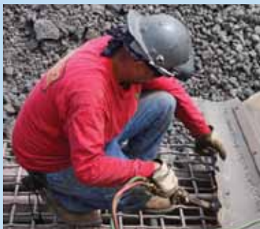
Welder Dewey Matsumoto repairs a scree while working on a new sewer plant.
