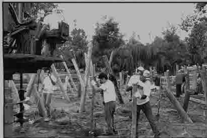
◀ As drill rig operator Erik Bakken of Viking Drillers bores holes, other volunteers place poles in preparation for construction of the playground's multi-level structure.
