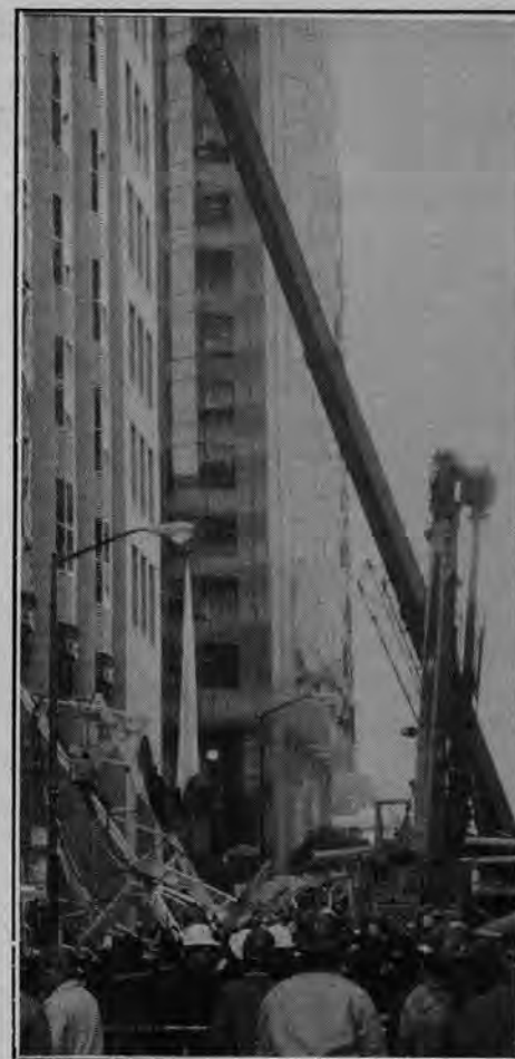
Sheedy moves in hydraulic crane to begin removing wreckage.
