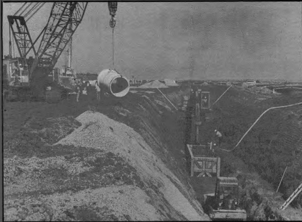
Granite Construction crew (above) excavates trench for storm drain.
