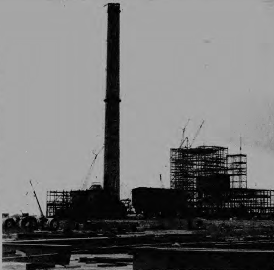
A 1982 photo of the Moon Lake power plant under construction.
