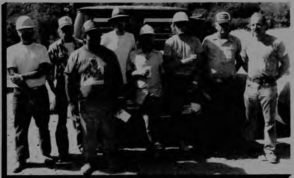
BACK WHEN THE WEATHER was a little warmer, this photo was taken of Plombo's crew working on the $1.4 million Geysers Road project. Pictured from left to right are: Jerry Nelson, John Davis, Richard Lawson, "Rollover" Steve Allen, Art Wisterman, Bob Martin, Dan Morton and John Valera.
