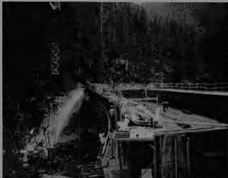
C.K. Moseman's project on the Smith River is comprised of two bridges, each containing about 1,800 yards of concrete and measuring 445 feet to 472 feet long. A 400-foot retaining wall is also in the works.
