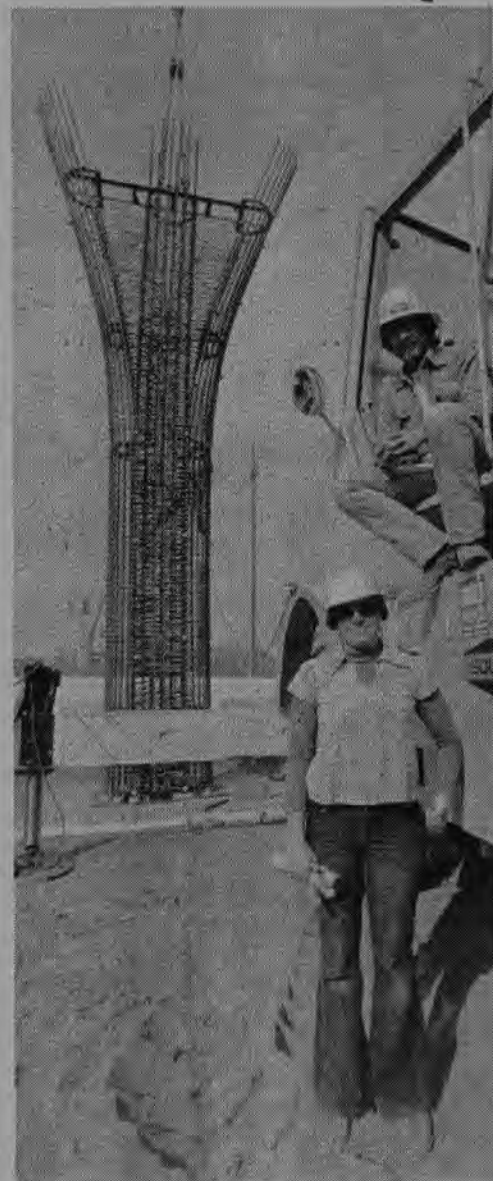
Operator Mike Darrough and apprentice Barbara Mooney are doing the steel work on the interchange project. Erecting falsework in the photo to the left are (left to right) Bud Lampley, Jr., Terry Garcia, David Eaton and Len Larson.
