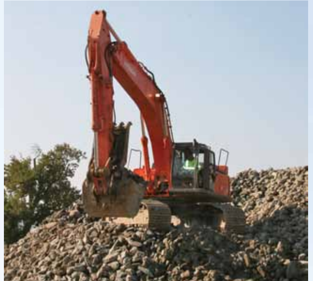
Excavator Operator Roman J. Serrano stockpiles the rock that has been removed from Grant Line Canal. It will be stored at this Howard Road/Tracy Boulevard rock storage location until April, when operators put it back in the river, so the pumps don't go dry.
