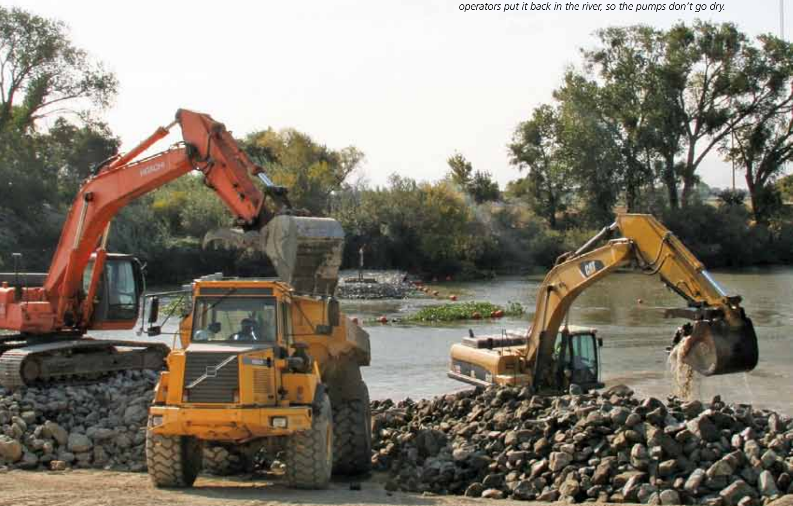
Excavator operators Greg "Hammer Hawk" Marino, left, and Norm Threlkel fill a haul truck operated by fourth-step Apprentice Opal Connor with rock pulled out of Grant Line Canal. Connor moved three loads of rock an hour on this 3,500-ton project.
