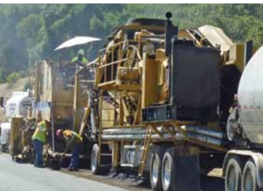
Members operate Pavement Recycling Systems' unique recycling machine, known as "the train."
