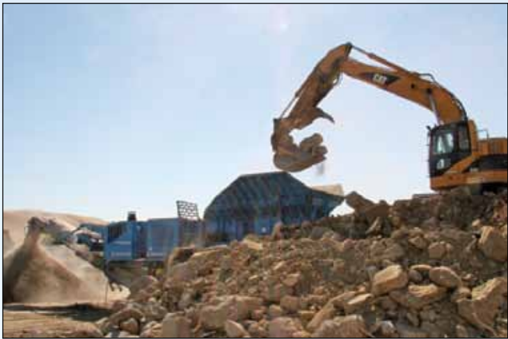
Excavator Operator Mario Giovannetti feeds the crusher to make roads for the Los Vaqueros Reservoir.
