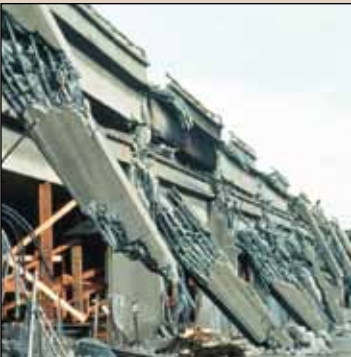
When the earthquake hit, the uprights that held up the top deck of I-880 separated and let the top deck fall.
