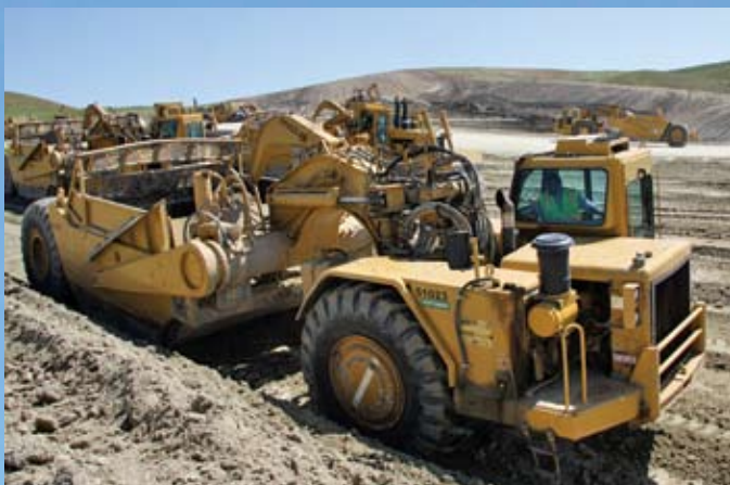
Operator Roman Rodriguez makes a cut with a 651 scraper and will pull about 35 yards on each run down the hill.
