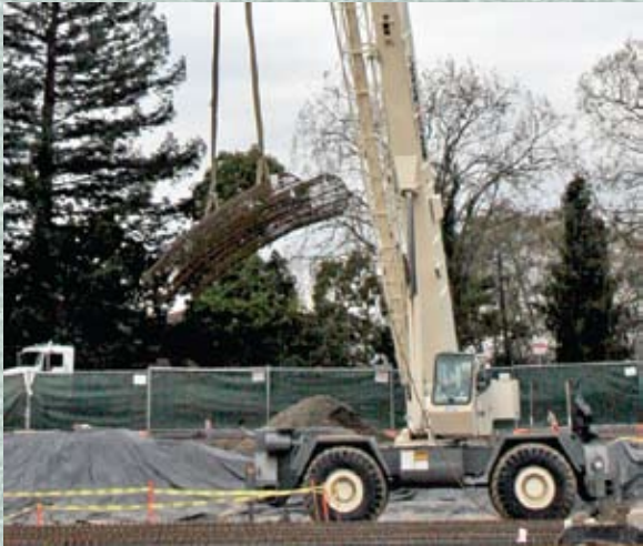
Crane Operator Daryl Hardy unloads cages with a 50-ton RT.
