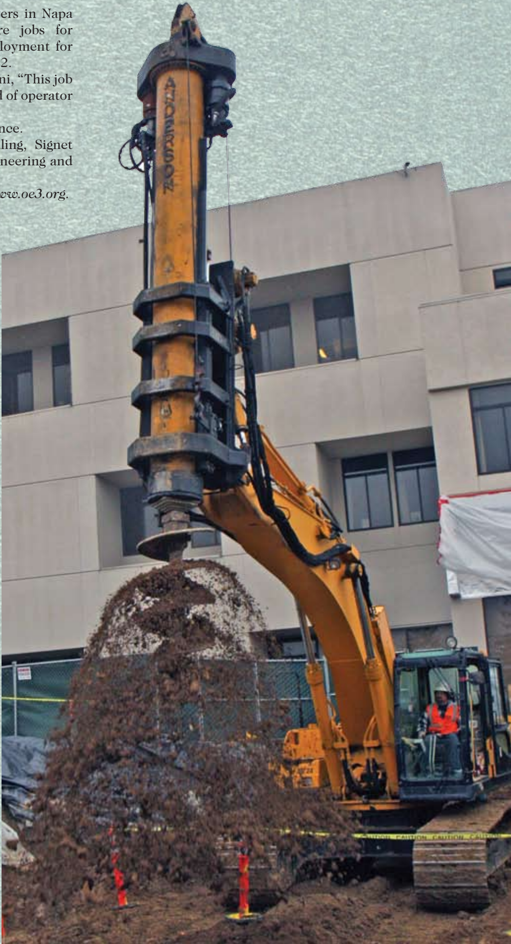
Lo-drill Operator David Harrigill removes spoils from the drill bit.
