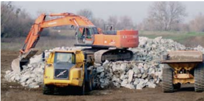
Cal-Neva crews repair part of a levee that broke in 1997.
