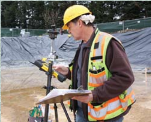
Surveyor Brian Tomlinson stakes the pilings for BKF Surveying.
