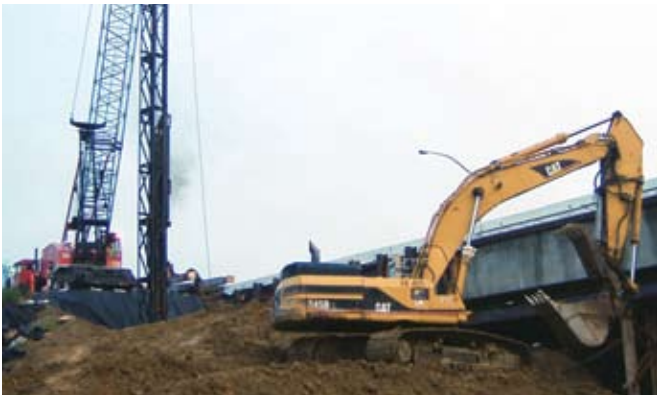
Gordon N. Ball excavates, while Cooper Crane drives pile.
