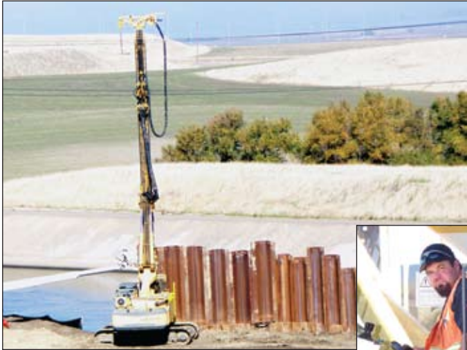
Eighteen-year member Ted Hughes operates the ABI pile driver.
