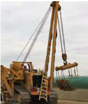
The lowering-in crew uses side booms to lift and lower the pipe into the ditch.
