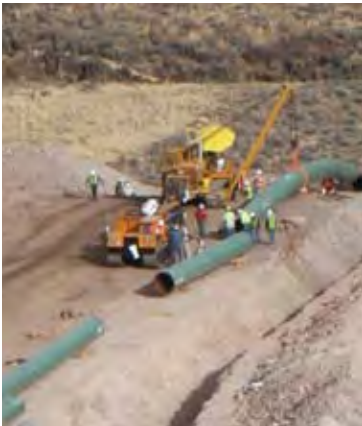
The bending crew slightly bends the pipe so it fits the contours of the land on the pipeline route.
