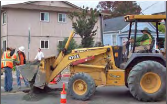
Backhoe Operator Rick Acosta potholes a storm drain.
