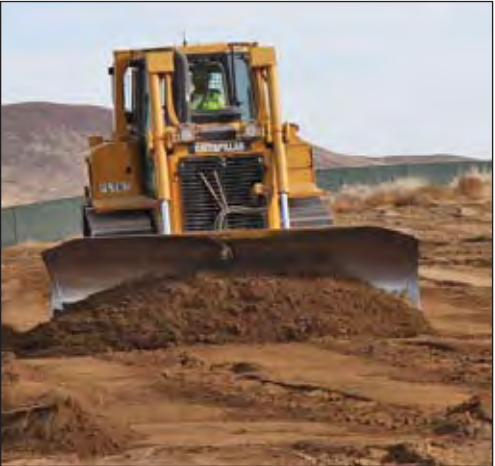
As part of his training in November, Floyd Bryant cuts the Right Of Way (ROW) down to grade.
