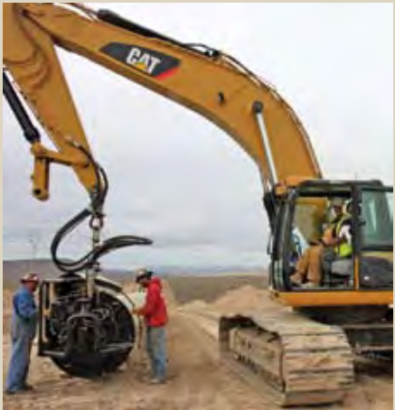
Jim Ryan's excavator is rigged up for end facing for automatic welding.
