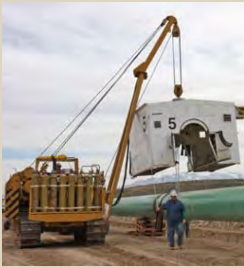
Pipe crewmember Ernie Gray moves a “tent” into position for the final cap. These tents protect the welders from the elements.
