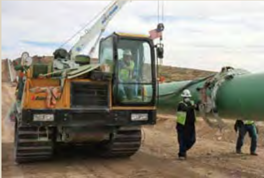
Coating crewmember Wade Grimm moves the flocking ring into position.
