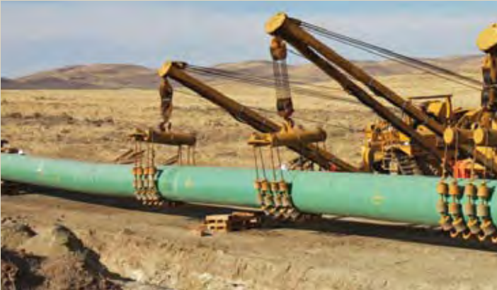
Lowering-in Foreman Blue King (also shown on the cover) rigs five side booms up Elko, Nev. King has made a career out of following the pipeline work. For more
