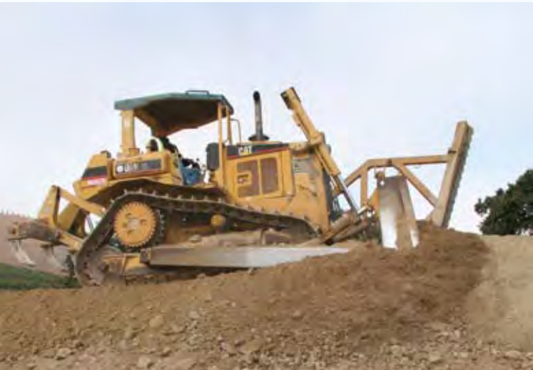
Seven-year member Brian Torri operates a D6 dozer with a slope board on the Hwy. 116 job in District 10.
