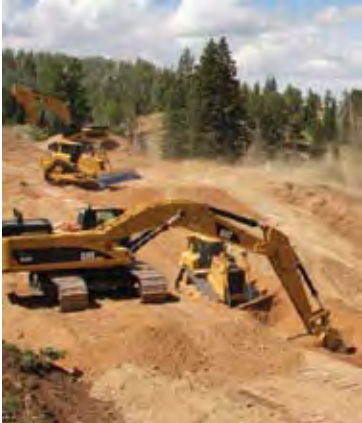
The ROW crew prepares a 115-foot-wide, level working surface for the construction equipment.
