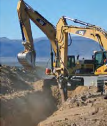
The ditch crew digs about 6 feet deep to make room for the 42-inch pipe.
