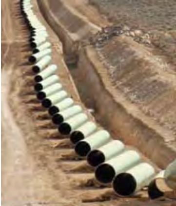
The stringing crew uses specialized trailers to move the pipe from the yard to the ROW, “stringing” it along the ROW.
