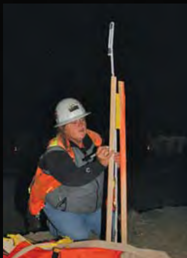
Gradesetter Sabrena Rosenberg sets grade at night along Hwy. 116.
