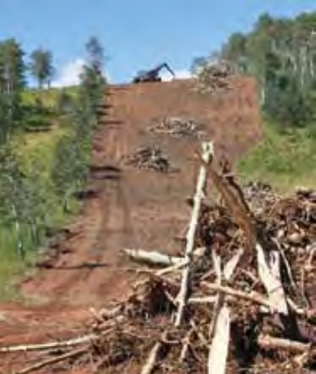
The clearing crew leads off by removing trees, boulders and debris.
