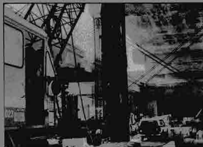
▼ Ian Ferguson, on a 2900 Manitowoc, drives pile along the Jerrold to Evans avenue section.
