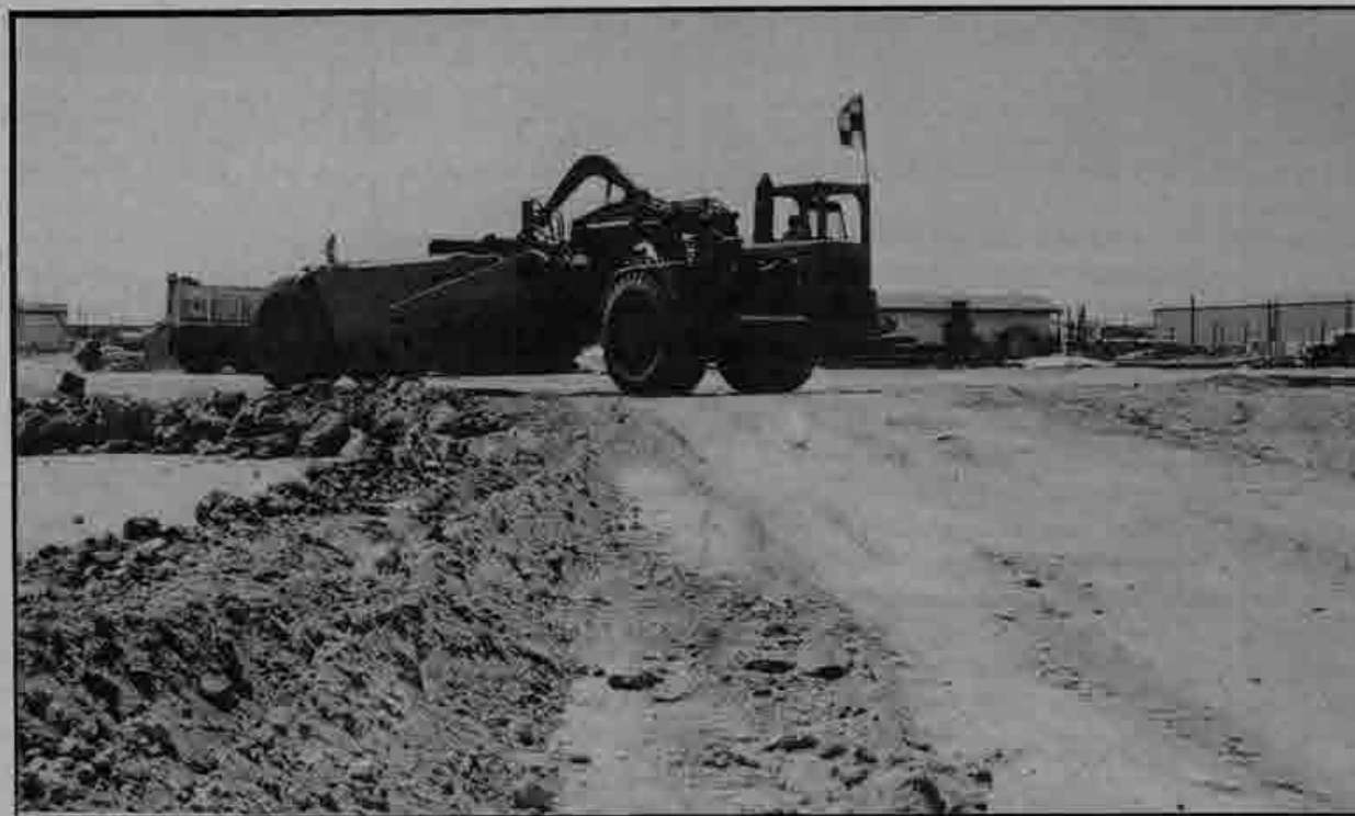
A scraper prepares to grab a load at construction of a huge aircraft maintenance complex in Tijuana.
