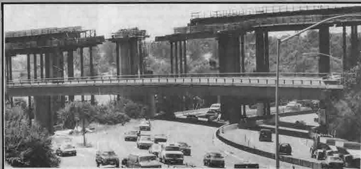
Right: A temporary bypass that has become the project's trademark rises above the I-680/Hwy. 24 interchange.
