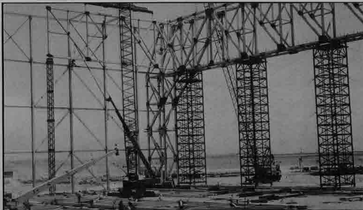
Erection crews place steel beams in place on one of the huge aircraft hangars at the new Tijuana maintenance facility. Under NAFTA, construction projects like this one will be built in Mexico rather than in the United States.
