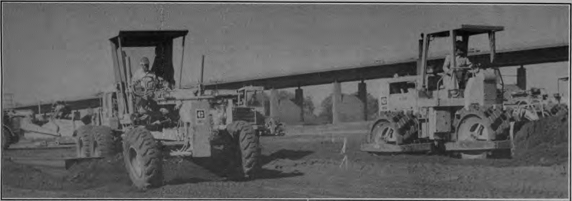
Local 3 members, delivering on a promise made last spring, volunteer their labor to help construct a new Riverfront Soccer Complex in Marysville.
