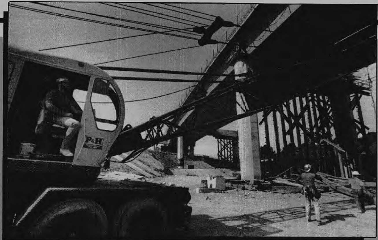
Apprentice Marlena Willis (left) assists operator Nick Moreno (above) in stripping forms.
