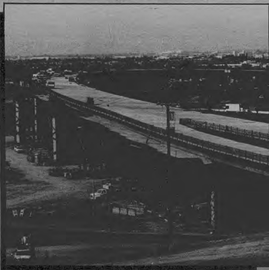
Major ramp on I-580 interchange nears completion.
