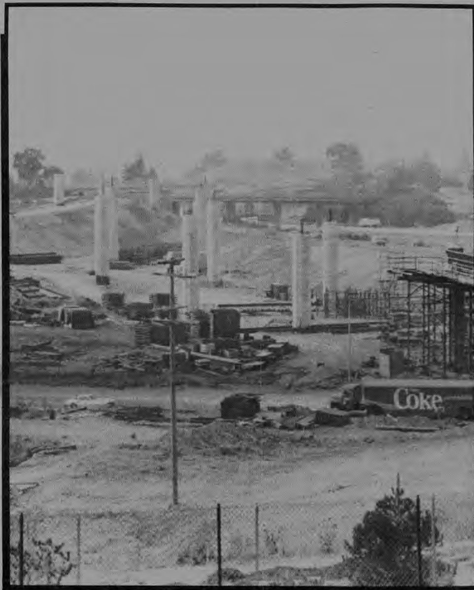
Equipment stands idle at I-580/Route 238 Interchange project.
