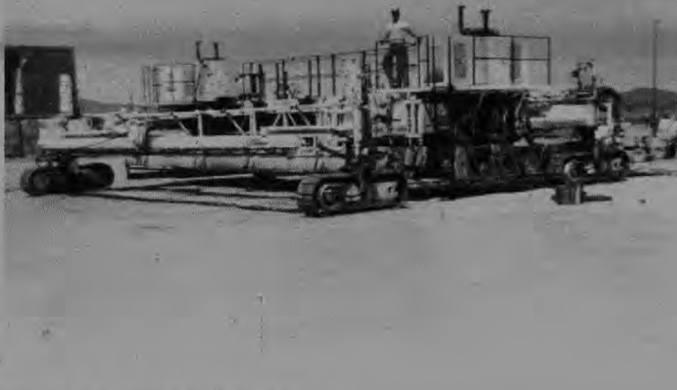
Operator Jim Woolstenhulm (above) moves the Guntert & Zimmerman paver on the I-15 job for James Cape & Sons near Beaver, Utah. To the right is a batch plant with two 12-yard mixers. Going full bore the crew was able to crank out 6,120 yards in a 12-hour shift.
