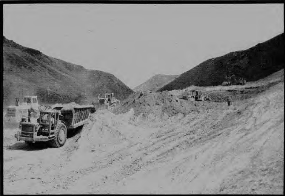
G-P Construction moves 150,000 yards of dirt on realignment and overlay of Carlin Gold Mine Road. Apprentice Jess Nachrondo (above) operates a compactor while rubber tired loader operator Mark Mosely stops to discuss a problem with Business Agent Derlin Proctor.
