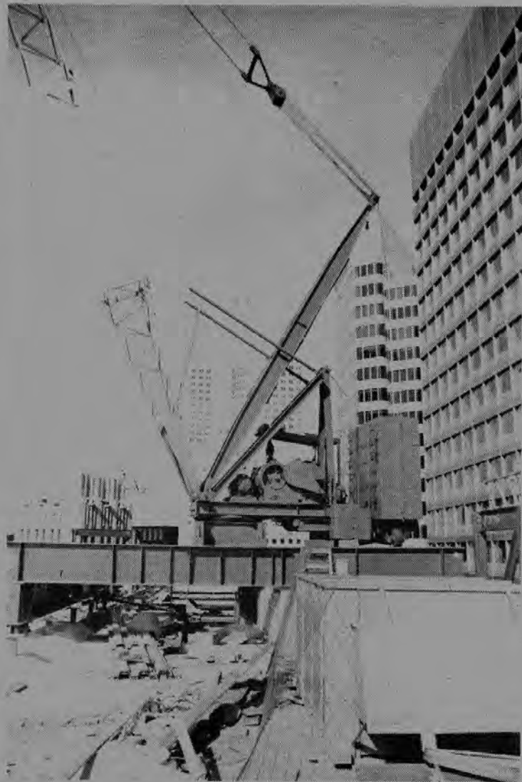
Bring in the ringer — It took a specially designed roof-mount ringer crane to make the heavy lifts on Dinwiddie Construction's First and Market Street project in downtown San Francisco. Made by Sheedy Crane, the ringer is mounted on top of the 28-story building. Because the weight of the stone panels were heavier than the normal lifting capacity of tower cranes, Sheedy had to design this special rig. The crane is equipped with a 46,200 lb. counterweight, 100-foot boom and 30-foot mast. It is capable of lifting 52,700 pounds at a 20-foot radius. Crane operator Bruce Maes is pictured at the controls.
