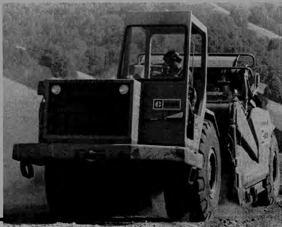
Pictured above, loader operator moves rip rap into the stream that will drain the man-made lake. Pictured lower left is mechanic Eddy Nave. Pictured far left is part of the housing complex that will contain the film facilities as well as corporate offices.
