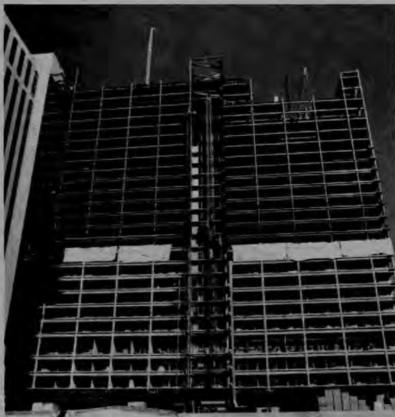
982-room additions to the MGM Grand-Reno PAGE 4/ENGINEERS NEWS/NOVEMBER 1980
