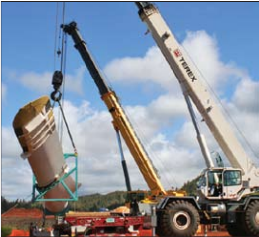
Terex Crane Operator Greg Scher of RMT and Alex Needham of American Piping & Boiler double-pick a blade for the windmill towers going up in the Kahuku hills.
