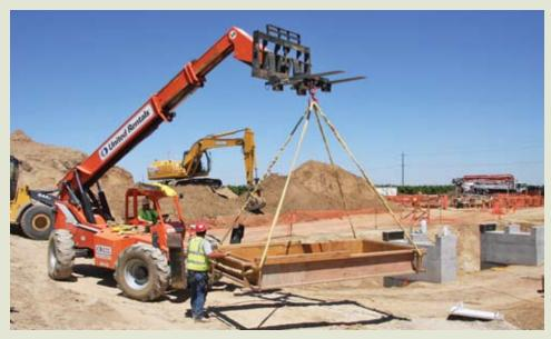
Forklift Operator Mike Darnall moves a form for a concrete pad as part of the compressor station.
