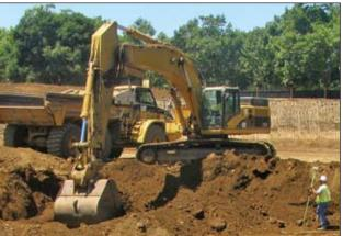
Excavator Operator Bruce Corey loads an ejector truck, while member Don Coronado uses GPS Rover to check grade.
