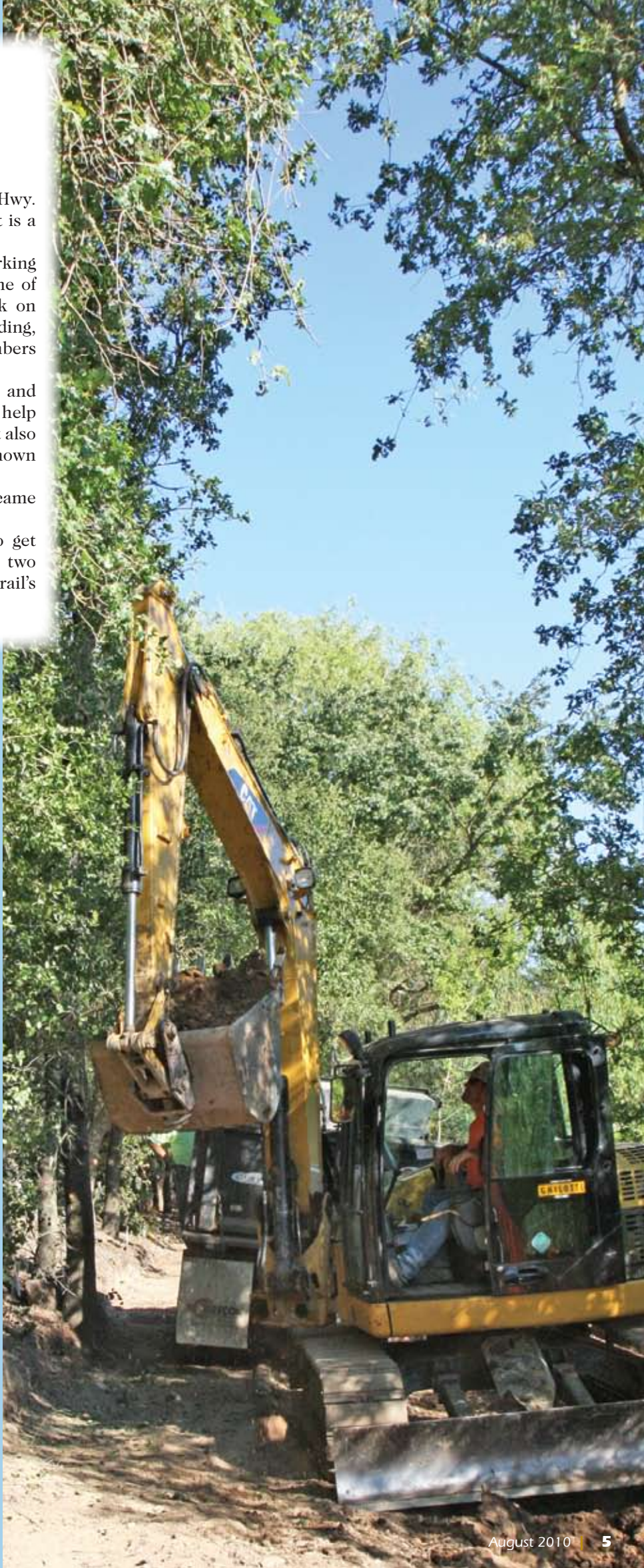
Bill Silacci maneuvers the bucket through a tight spot as he digs the trench for one of the walls.
