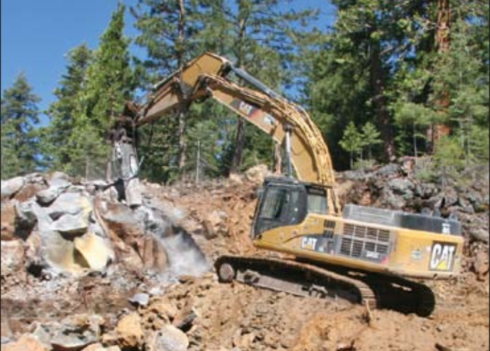
Hoe-Ram Operator Leon Johnston breaks up rock to be hauled away.
