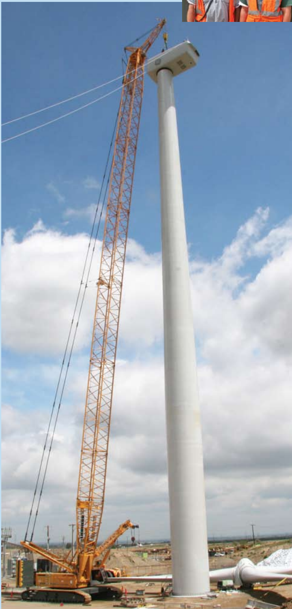
Crane Operator Bill Alger hoists the nacelle to the top of the windmill's tower. The nacelle is the energy-producing part of the structure, as it contains the gear box, low- and high-speed shafts, generator, controller and brake. This process took about 45 minutes to complete.
