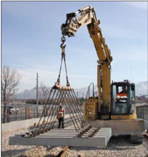
Jake Carlson lays ties for the new light-rail line.
