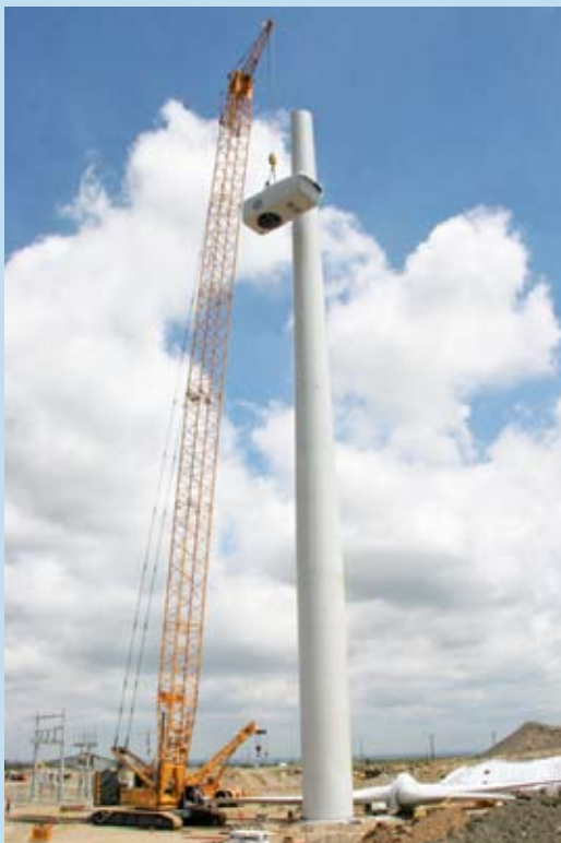
Crane Operator Bill Alger hoists the nacelle to the top of the windmill's tower. The nacelle is the energy-producing part of the structure, as it contains the gear box, low- and high-speed shafts, generator, controller and brake. This process took about 45 minutes to complete.
