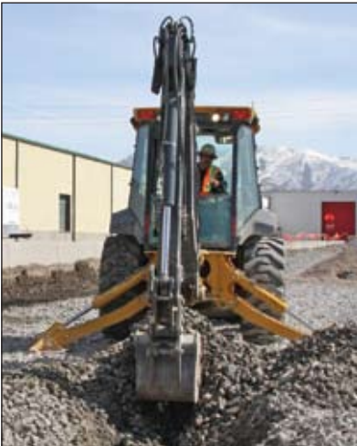
Tim Squire makes cuts for communication and power.
