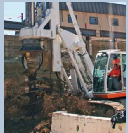
Drill Operator Michael Powell drills 55-foot holes for the cages and eventual piers.
