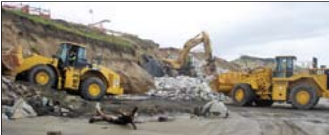
Operating Engineers Chris Giordino, Randy Davidson, Joe Alfaro, Rich Carrilla and Jason Enna place rip rap at Ocean Beach in San Francisco for Ghilotti Bros. Construction.
