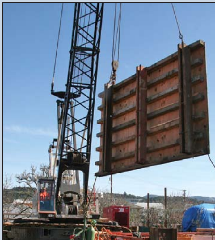
Kiewit Crane Operator Randy Silva strips concrete panels.
