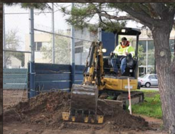
Six-year member Joe Silva cuts grade for the new Eastridge Little League walkway, working carefully under and around a tree that needs to be saved.
