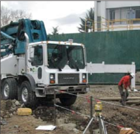
Conco Pump Operator Augustin Hernandez sets up an outrigger as he prepares to pump concrete.
