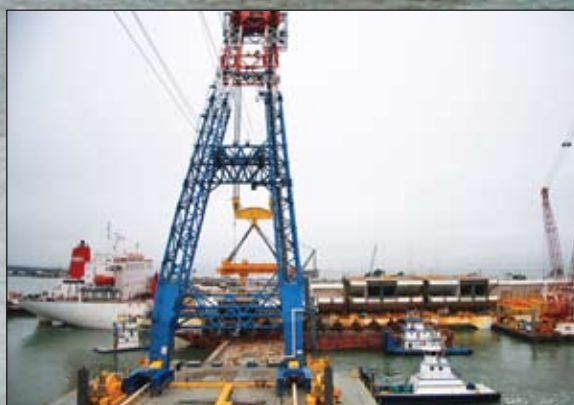
The Hero holds the Left Coast Lifter in place while Eventide positions the barge under the 800-ton section.
