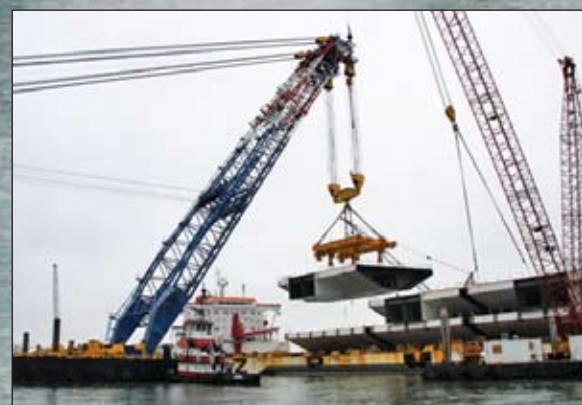
The second section, weighing 800 tons, is lifted off the ship.
