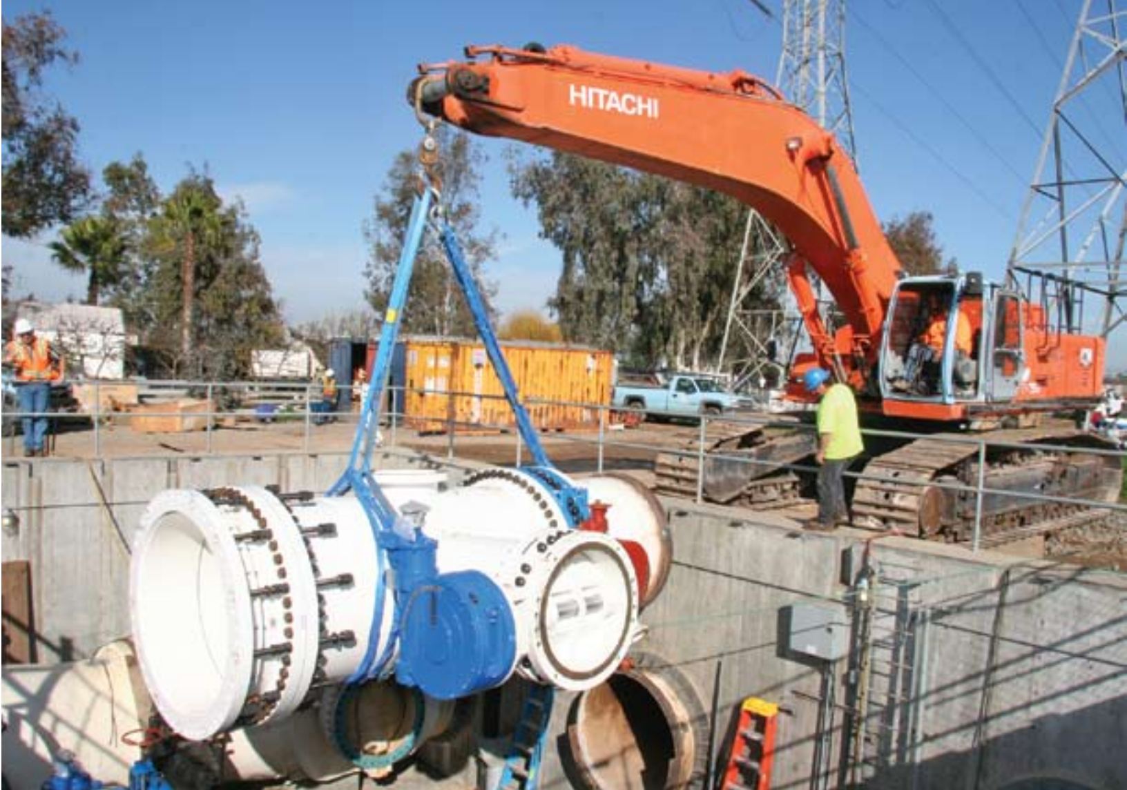
Operators Mark Alire and Scott Ross work together to steady and lower a 38,000-pound valve east of Salida in Riverbank. This replacement is one of three for the Hetch Hetchy Water System Improvement upgrades.
