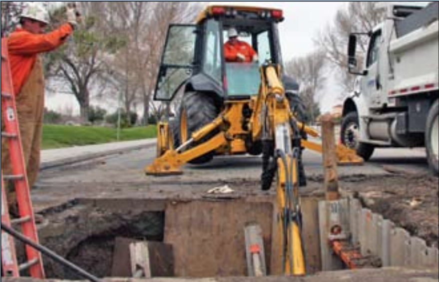
Rich Green uses hand signals to help Backhoe Operator John Horry dig to an existing waterline they will tie into.
