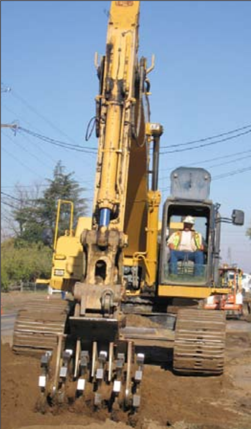
Excavator Operator Arron Cline compacts the trench.
