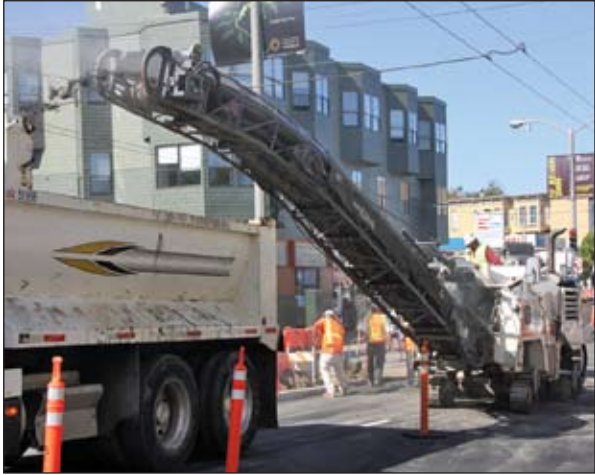
Members working for ABSL Construction grind out sections of Divisadero Street.
