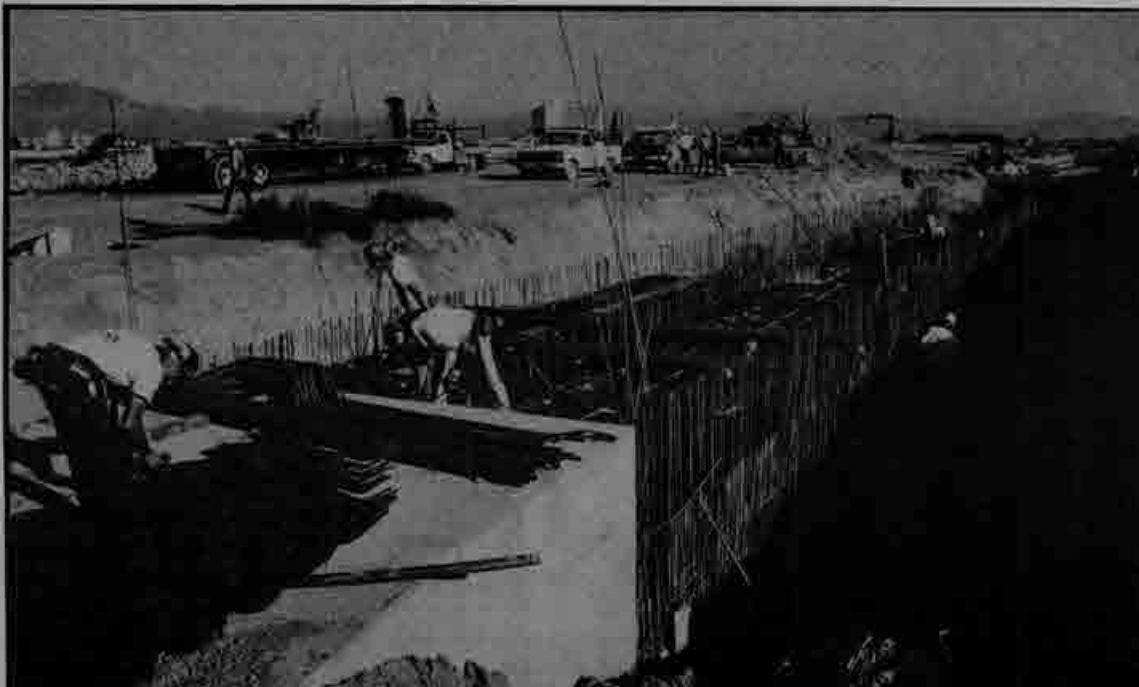
Bottom left: Drainage improvements such as this box culvert, are a major component of Reno's runway upgrade.
