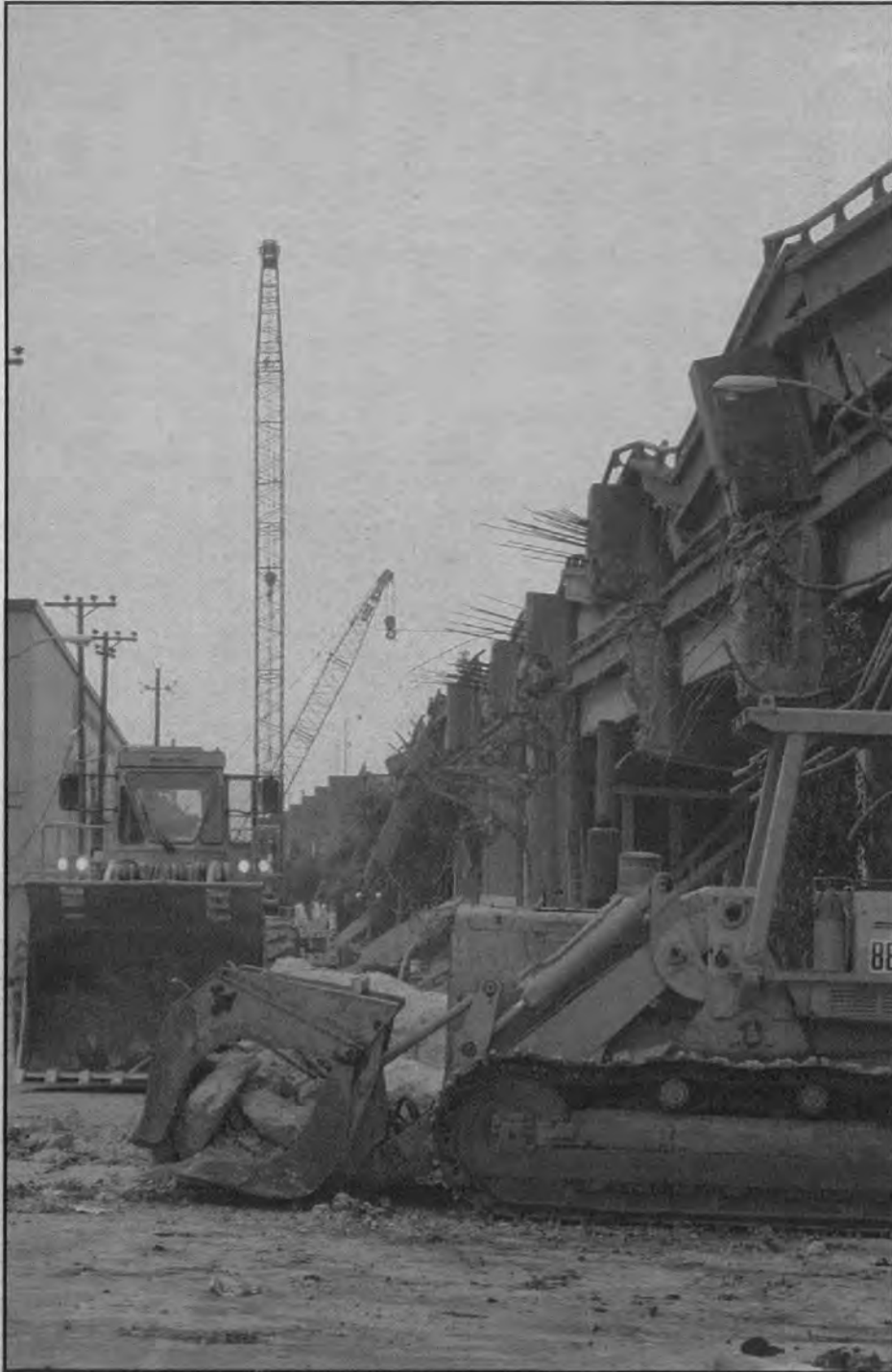
Loader operator for Oliver deSilva works with dozer to clear rubble at the collapsed Nimitz Freeway. Cranes in back belong to Bigge and MCM.
