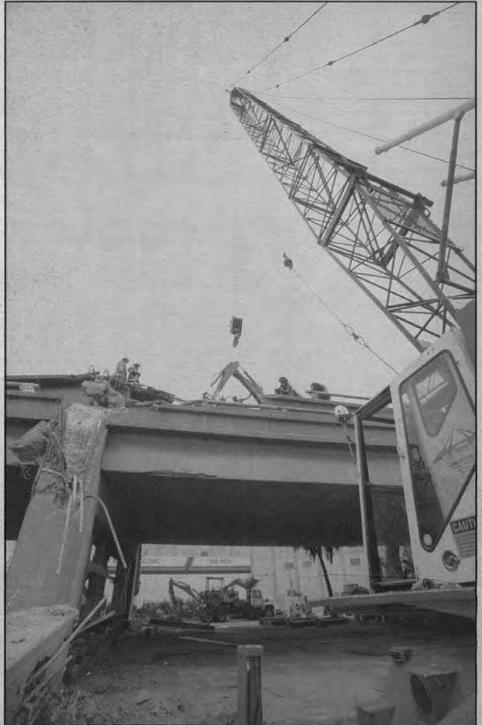
Crane operator Evan Trujillo of MCM Construction lifts concrete slab off of car buried under the freeway's upper deck.
