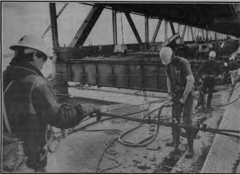
After concrete has been cut with saw, workers widen the gap with jackhammers to expose rebar below.
