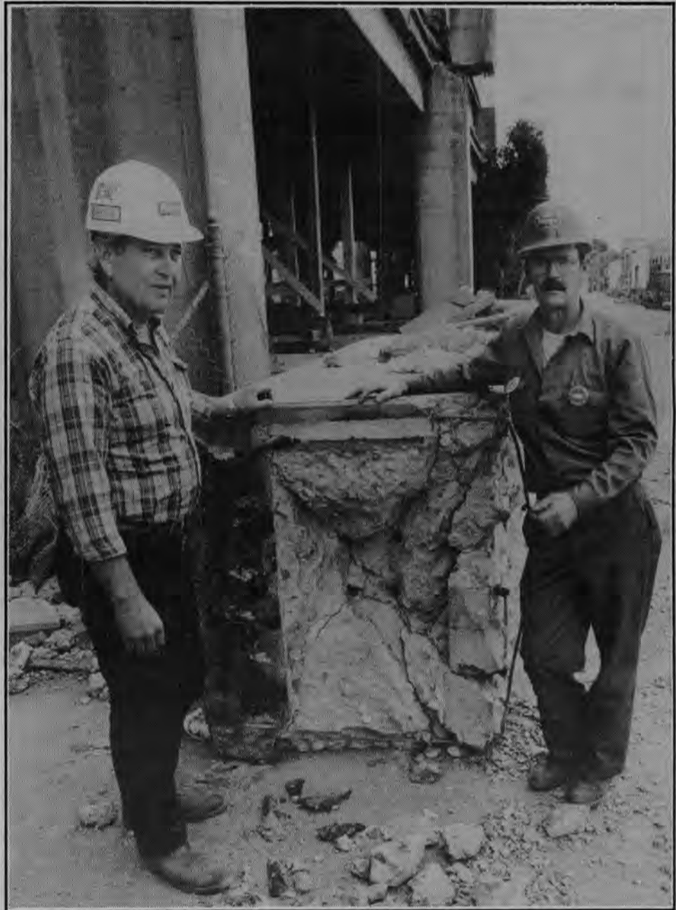
Operator Randy Burke (left) and Oiler Jay Brown of Bigge Crane point out the inadequa-
