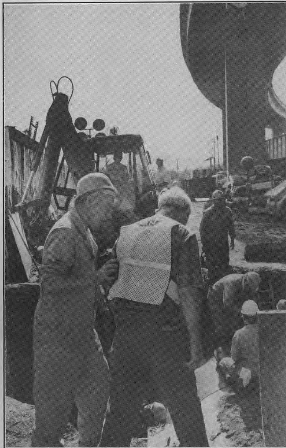
Mike Coccellato, an 18-year member, operates a Case backhoe for the Dept. of Public Works in San
