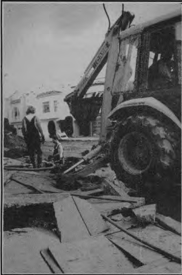
George Ballardo (left) runs backhoe during repair work in San Francisco's severely damaged Marina District. Local 3 backhoe operator Chris Kieselbach (right) assists emergency repair work on a broken water main on Pier 23. Sid Usry (below), assisted by his son Brian, operates Bigge crane at collapsed section of Nimitz Freeway.
