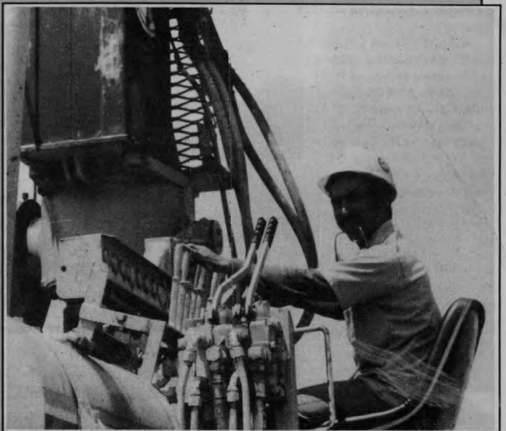
Mario "Mac" Casa, Jr. (above) operates drill for Kiewit. Pictured far left is Tim West, backhoe operator for Dan Caputo.
