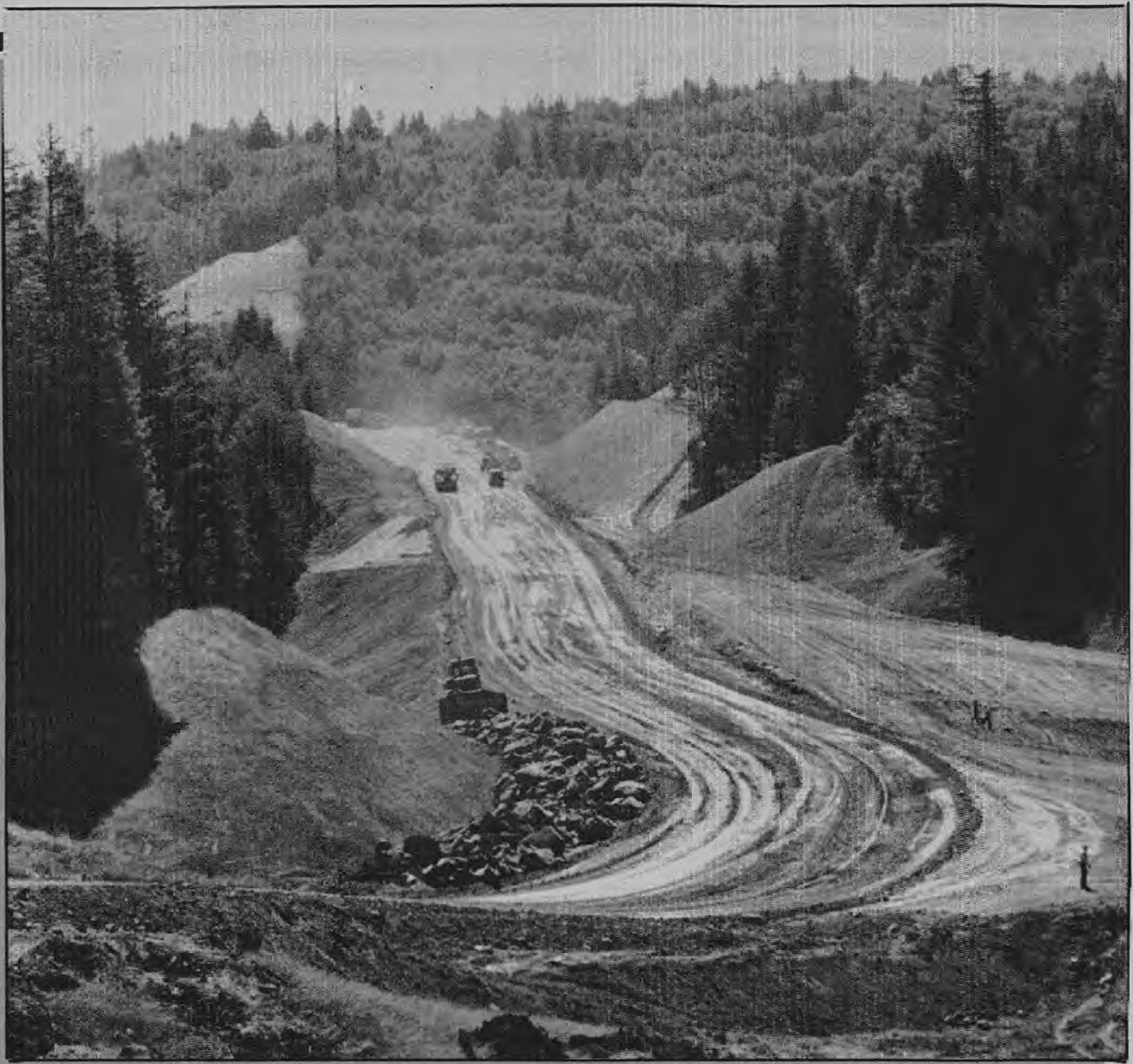
Tutor-Saliba's $67 million portion of the Redwood Bypass begins to take shape as they wrap up their second year on the job.
