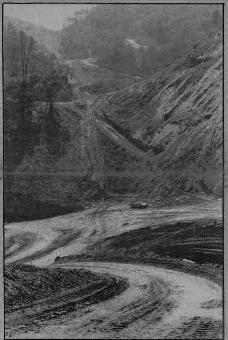
The first phase of the Cloverdale Bypass (above) is part of over $1 billion of work that has gone to Local 3 members as a result of project agreements.
