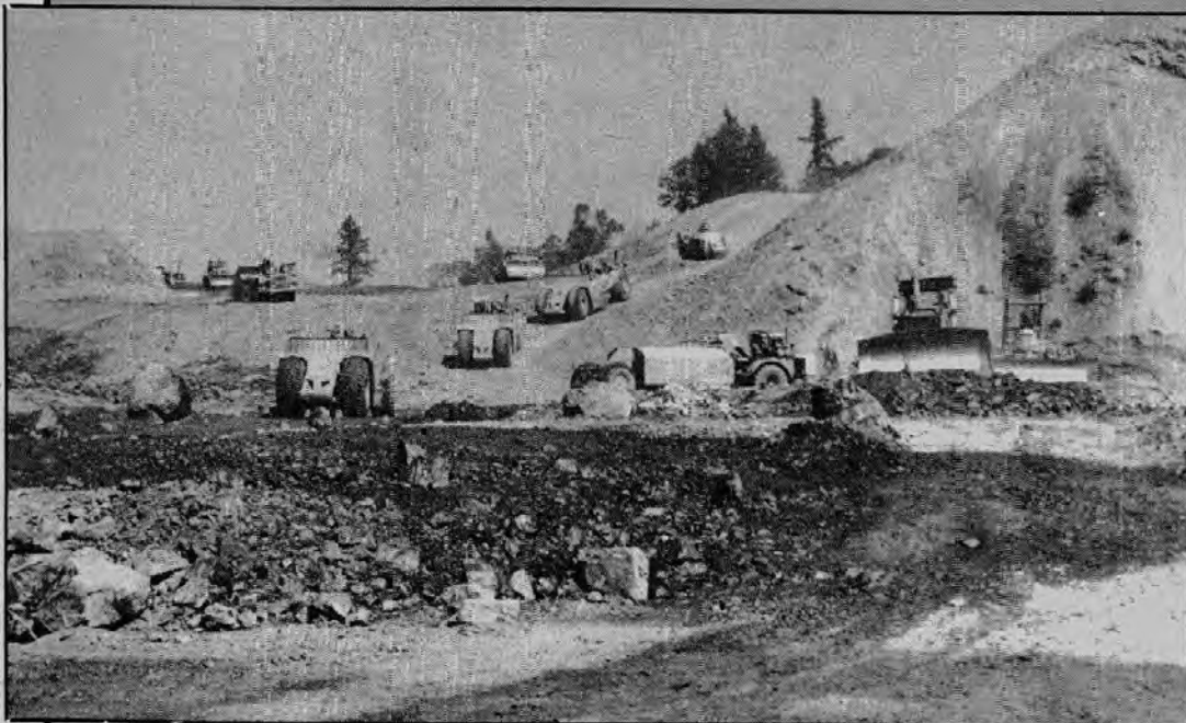
Local 3 operator (above) make one of many large cuts on Guy F. Atkinson's portion of the job. At right is mechanic Ralph Warts.
