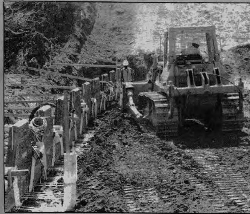
At left is mechanic Tony Cerna. Dozer operator Randy Alexander (above) assists workers in laying reinforced wire mats.
