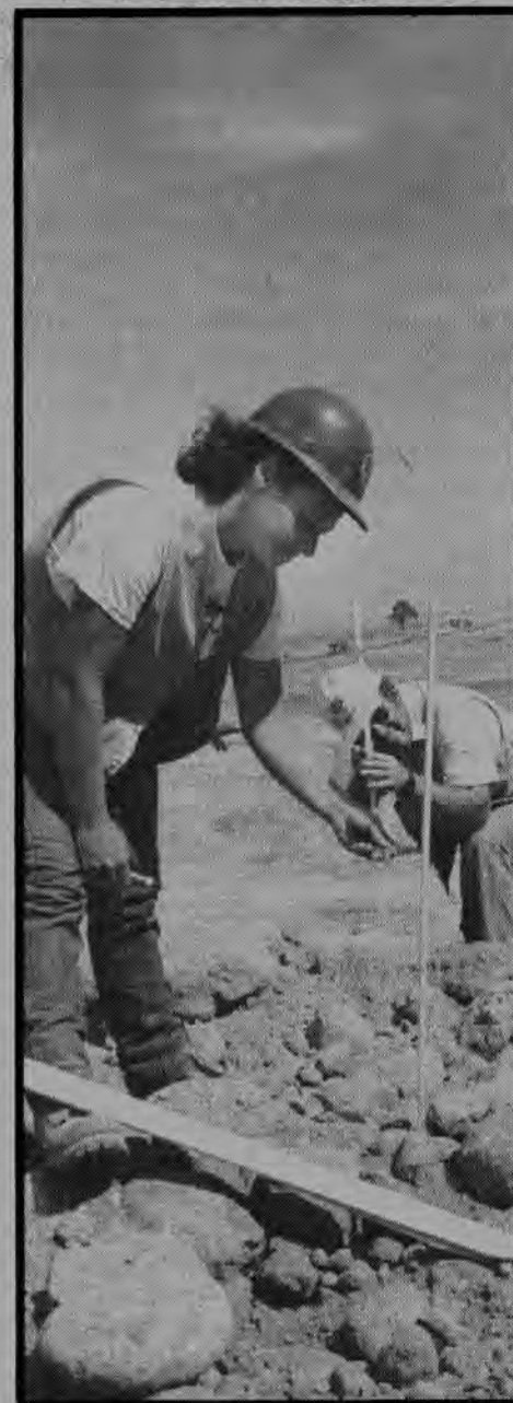
Gradechecker Bill Butler and apprentice Susan McFadden check grade on Granite Construction's job on Hwy. 65 near Roseville.
