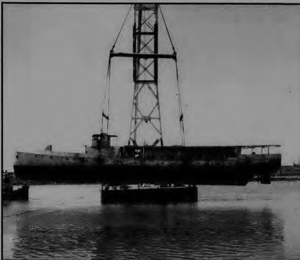
Manning Peter Klewit & Sons' 'Jan B' and rigging donated by Smith-Rice Company, Local 3 members lift the ailing Potomac from the Bay to begin restoration efforts.
