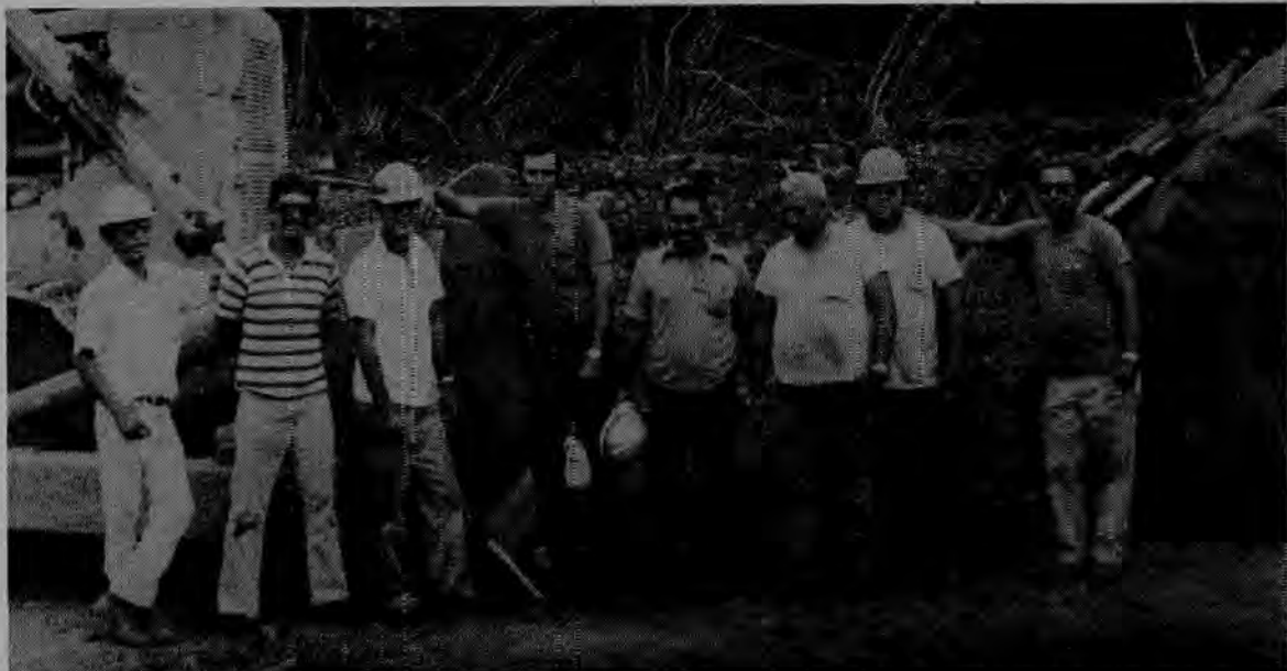
Operating Engineers working on the Panewa flood control project are (left to right) Jits Lawrence, Joe Velez, Joe Kuanoni, Tony De Sa and Allen Ahn. The job is being carried out by Sonomura Contracting.
