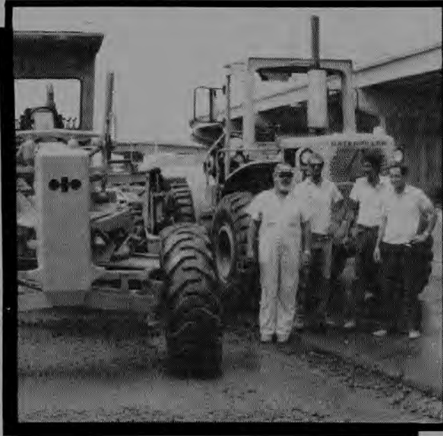
Pictured left is Hawaiian Dredging's airport viaduct project. Left to right are grader operator Ramon West, gradechecker Jim Merritt, loader operator Mike Nakanishi and foreman Ron Hall.
