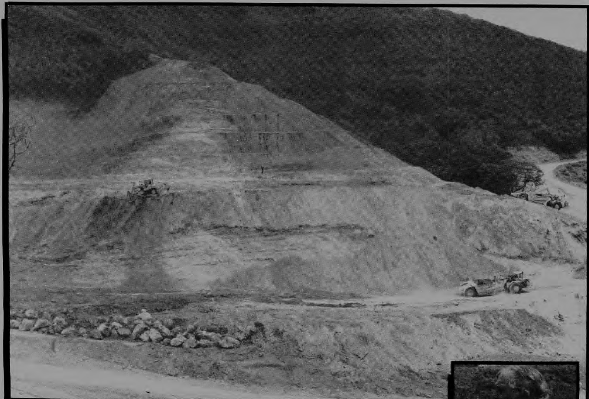
Pictured above is the Kailua landfill job underway by Highway Construction Company.
