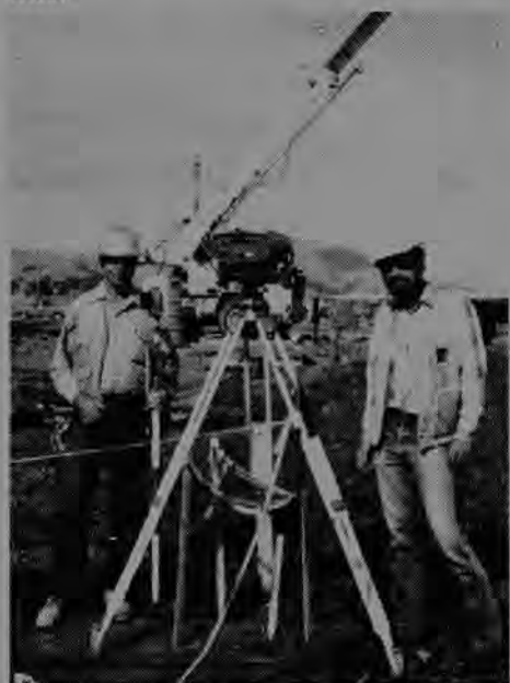
Pictured from left to right are John Prentice and Don Philips working in San Ramon on the P.T. & T. Building.
