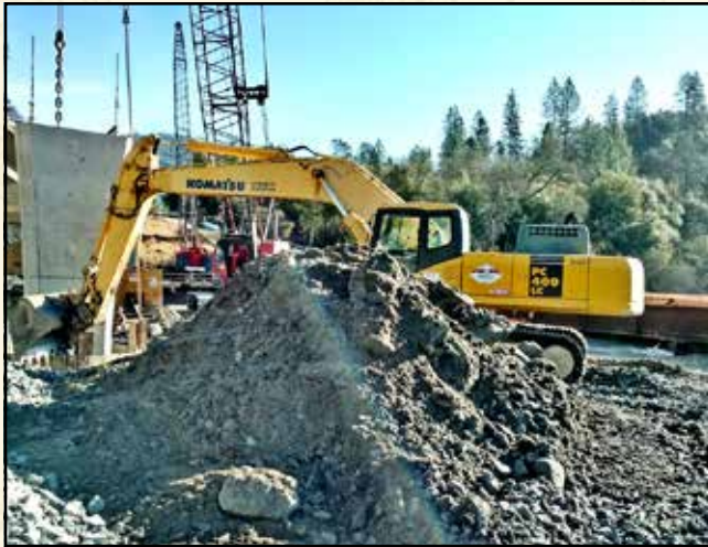
Excavator Operator Dustin Loftis works on a new bridge in Coloma for MCM Construction, Inc.
