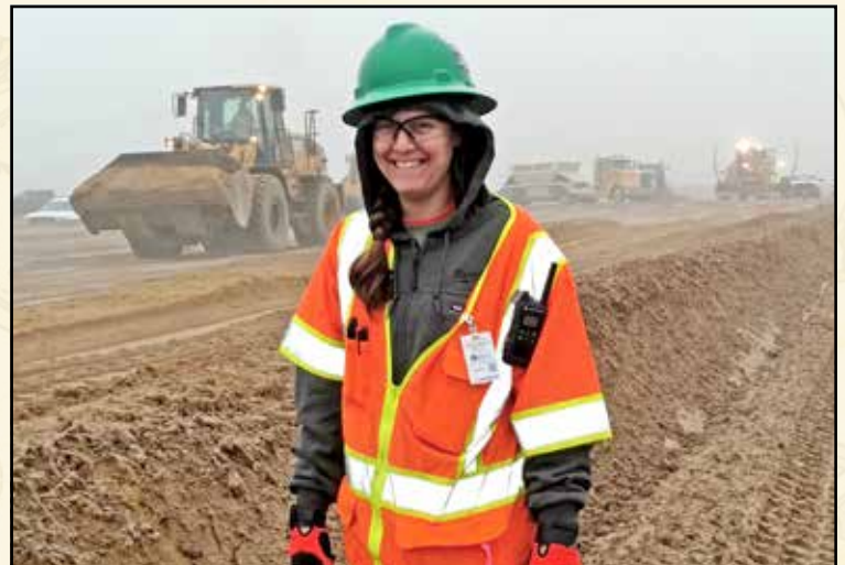
Member Jonell Murphy works on HSR for Dragados/Flatiron JV.
