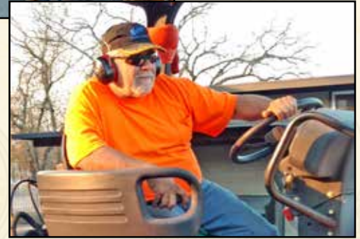
Roller Operator Kerry Long works on a church parking lot for Siri Grading & Paving.
