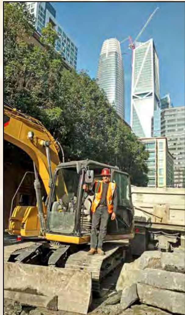
A. Ruiz Construction Operator Antonio Gonzalez installs new high pressure and domestic water mains in the Transbay District.
