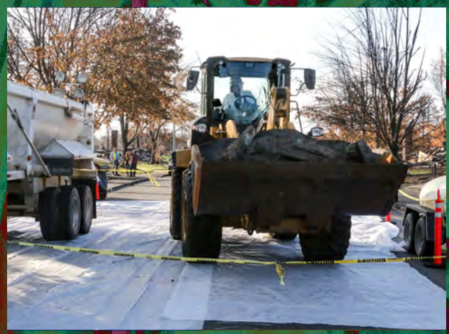
Operators like this one from Anvil Builders, must load trucks from the fire cleanup sites on tarps.
