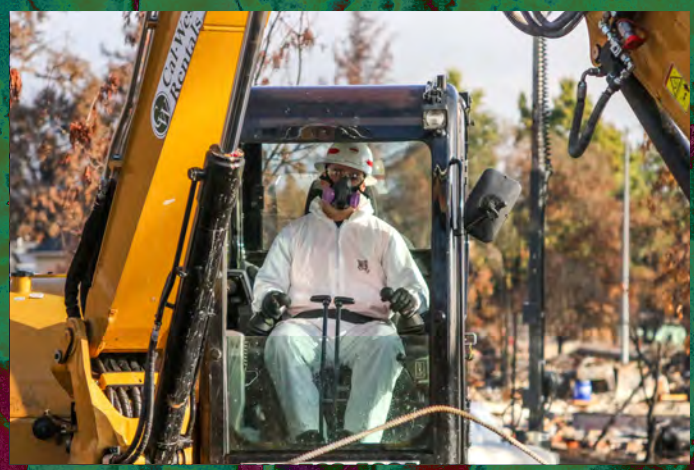
Excavator Operator Steve Nicholas loads up a truck with wreckage from the fire in Coffey Park.
