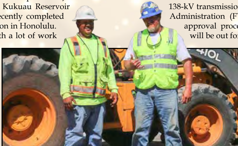
From left: Ron's Construction Foreman Vince Rabago and Operator Dennis O'Brien work on the Costco gas station project in Honolulu.
