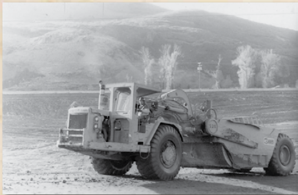
In 1988, the long-awaited Jordanelle Dam project gets underway as part of the Central Utah Project.
