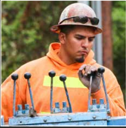
Malcolm Drilling Operator Cesar Zepeda drills for a shoring system on Hwy. 101 in Big Lagoon.
